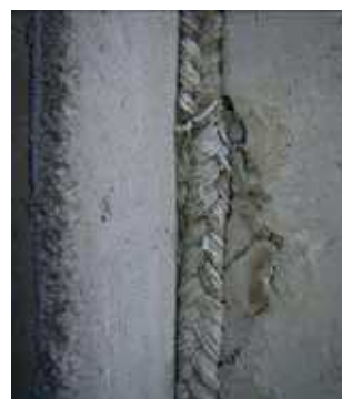
Joints de dilatation
